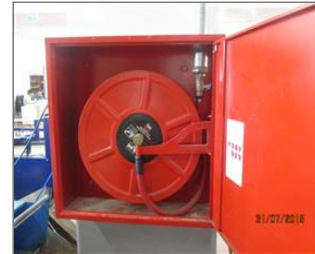
Photo of the inside of the main production hall IMG_2597.JPG
