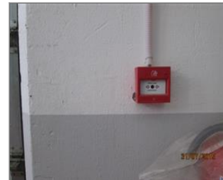
Photo of the inside of the main production hall IMG_2566.JPG
